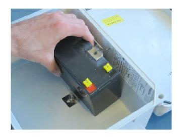
4) To install the new battery, follow steps 1–3 in reverse. Make sure the metal bracket that holds the bottom of the battery is flush against the battery before tightening. Do not over-tighten nuts.
